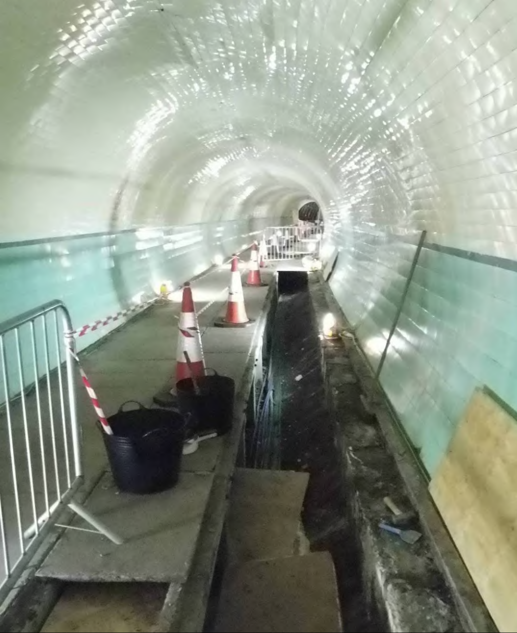
Paving flags in the Cyclist Tunnel have been lifted, to establish the route of much of the mechanical and electrical services for tunnel systems
