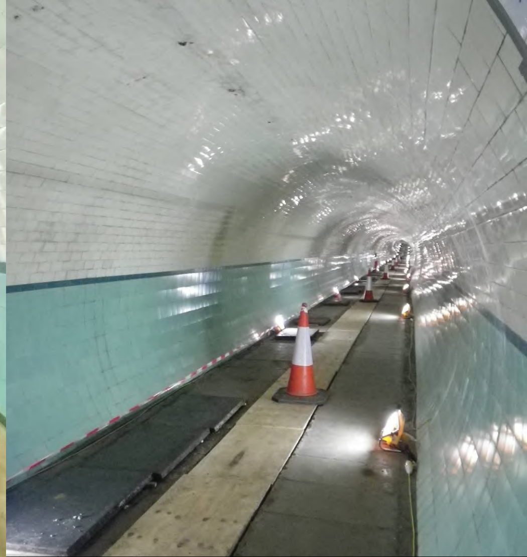
Ceramic tiles have been cleaned in both tunnels prior to repair of damaged tiles and re-grouting. Sections of flooring in the pedestrian tunnel have been removed for renovation/replacement. All the existing light fittings have now been removed.
