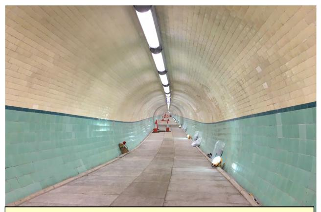
Hundreds on new paving flags have had to be manufactured for incorporation into the tunnels. The new paving flags have now been laid in place. The cyclist tunnel is complete and the contractor is well on with the paving works in the pedestrian tunnel.
