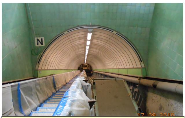
The scaffolding in the incline has now been removed to allow the inclined lift car to be completed. This will involve installing the glass walls and roof.
