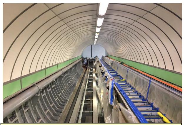
The tunnel lining has now been sealed, electrical and mechanical systems installed and the cladding panels renewed. The new inclined elevator installation is ongoing.
