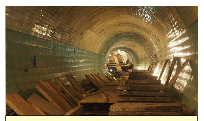
The tunnel paving has been lifted and relayed a number of times during the project to allow installation of new mechanical and electrical systems, to deal with structural repairs and asbestos removal.
