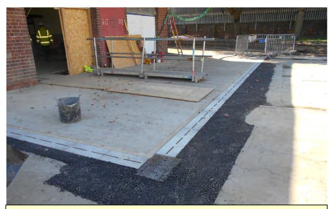
The concrete slab in from of the rotunda building has now been replaced as has the drainage. The next element of works externally is the replacement of the surfacing.
