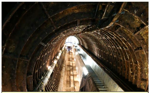
The refurbishment works required the removal of one escalator at each end of the tunnels and complete removal of the cladding system
