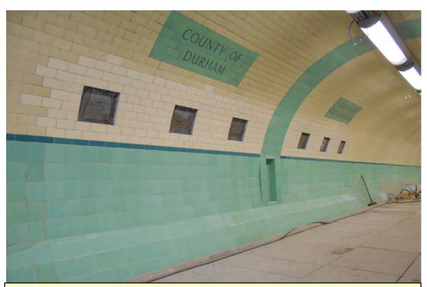
Following the installation of the new ventilation ducts the tiling has been replaced and only the duct covers remain to be installed.
