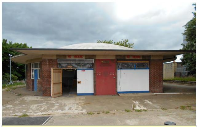
The external fabric of the rotunda buildings is being repaired and cleaned up. The concrete slab in front of the building has had to be fully replaced.
