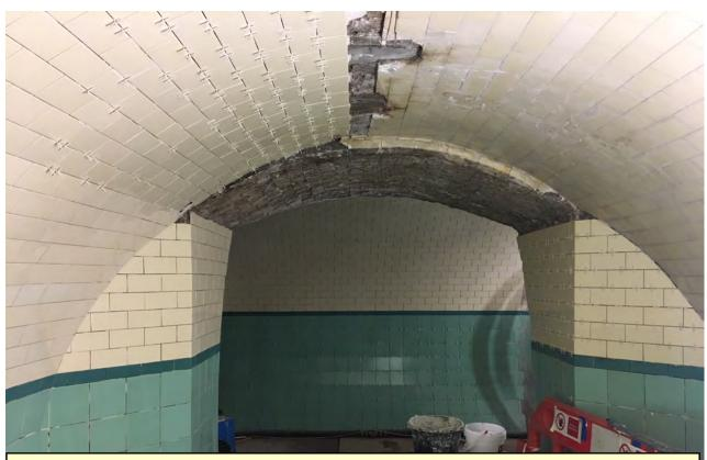
Once the tunnel leaks had been sealed new tiling has been laid. The tiles have been manufactured to match the existing tiles and are installed by heritage trained tilers.
