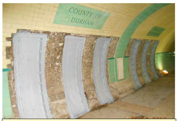
The ventilation ducts in the centre of the tunnel had to be completely replaced.
