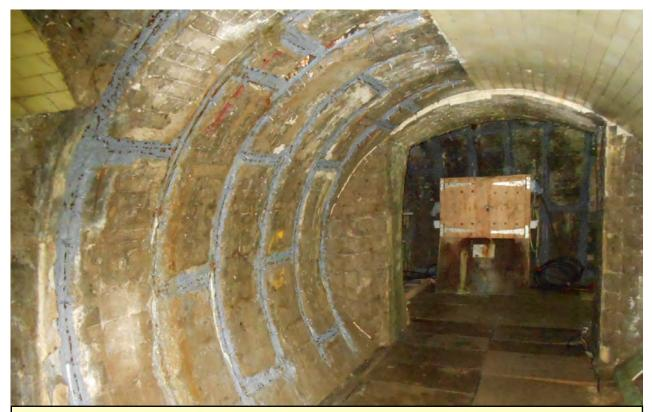
To deal with seepage into the tunnels large areas of tiles had to be removed and 'leaks' injected with resin to seal them.
